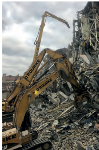
O'Rourke Wrecking Company climbed 13 places to 60th during 2019
