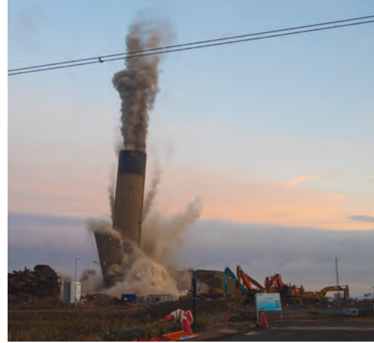
Brown and Mason proposed a vertical collapse mechanism for the Littlebrook chimney
